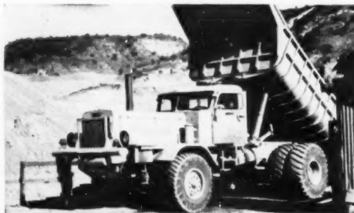
Buda powered Dart dumping at the crusher.
